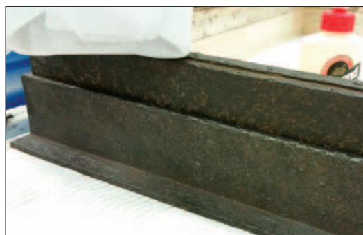
The base frame has been turned on its side, ripped to create an extender for the top capped moulding to rest upon.
