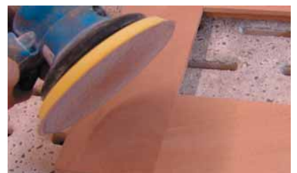
The frame is sanded flat using an air-powered sander. This also removes any remaining glue and milling marks.
