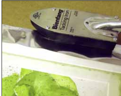
Wrap matte side of film to ATG tape, shiny side out. Note the outer edge shows the film has been melted to the tape.
